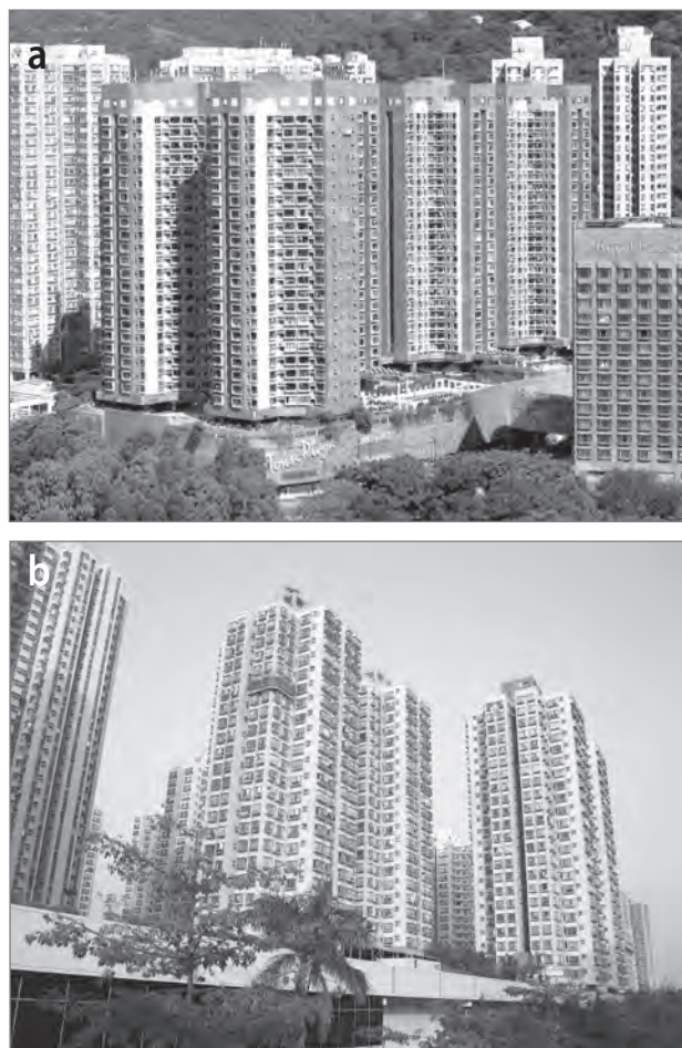
Figure 1: a) New Town Plaza in Shatin, b) Tai Po Centre in Tai Po (photo: Yung Yau).
