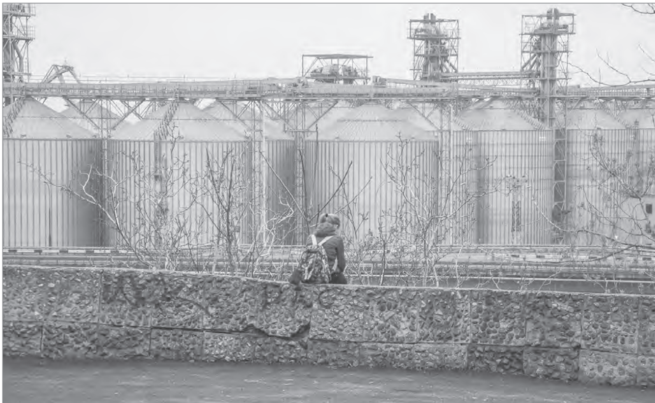
Figure 6: Construction of grain terminals in the centre of Odesa (photo: Stanislav Gref).
