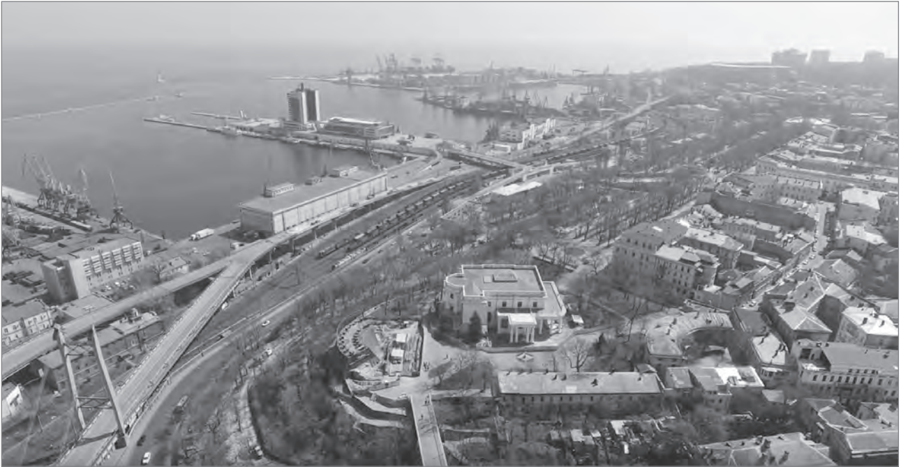
Figure 5: The new pier and Primorsky Boulevard (photo: Vladimir Khalin).
