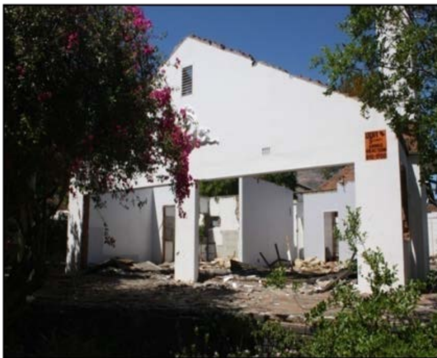
Photo 1: Example of a historic house that has been destroyed by vagrants (source: Authors)
