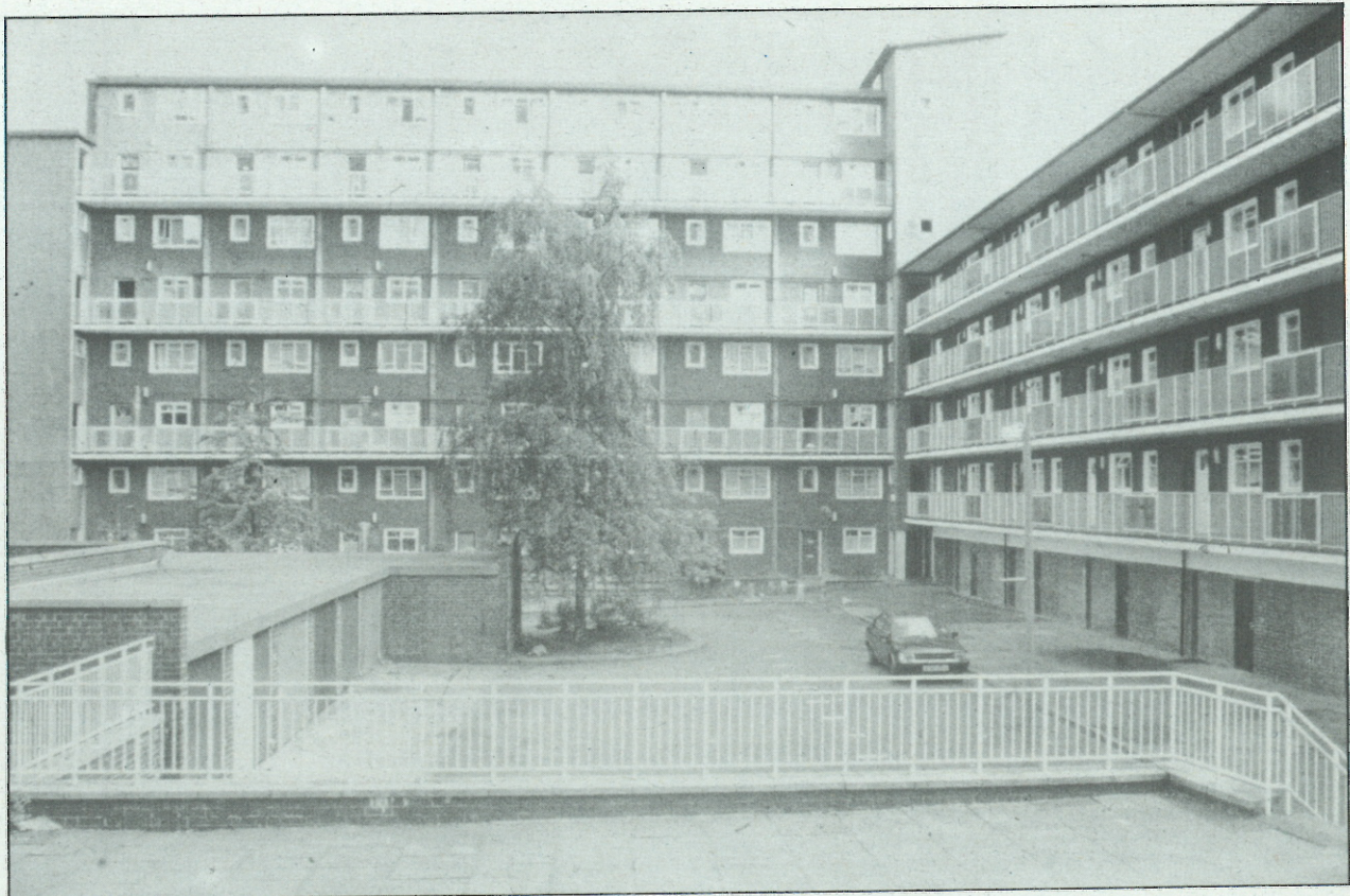
Picture 7: 1959 maisonette blocks about to be demolished in the Housing Association redevelopment
