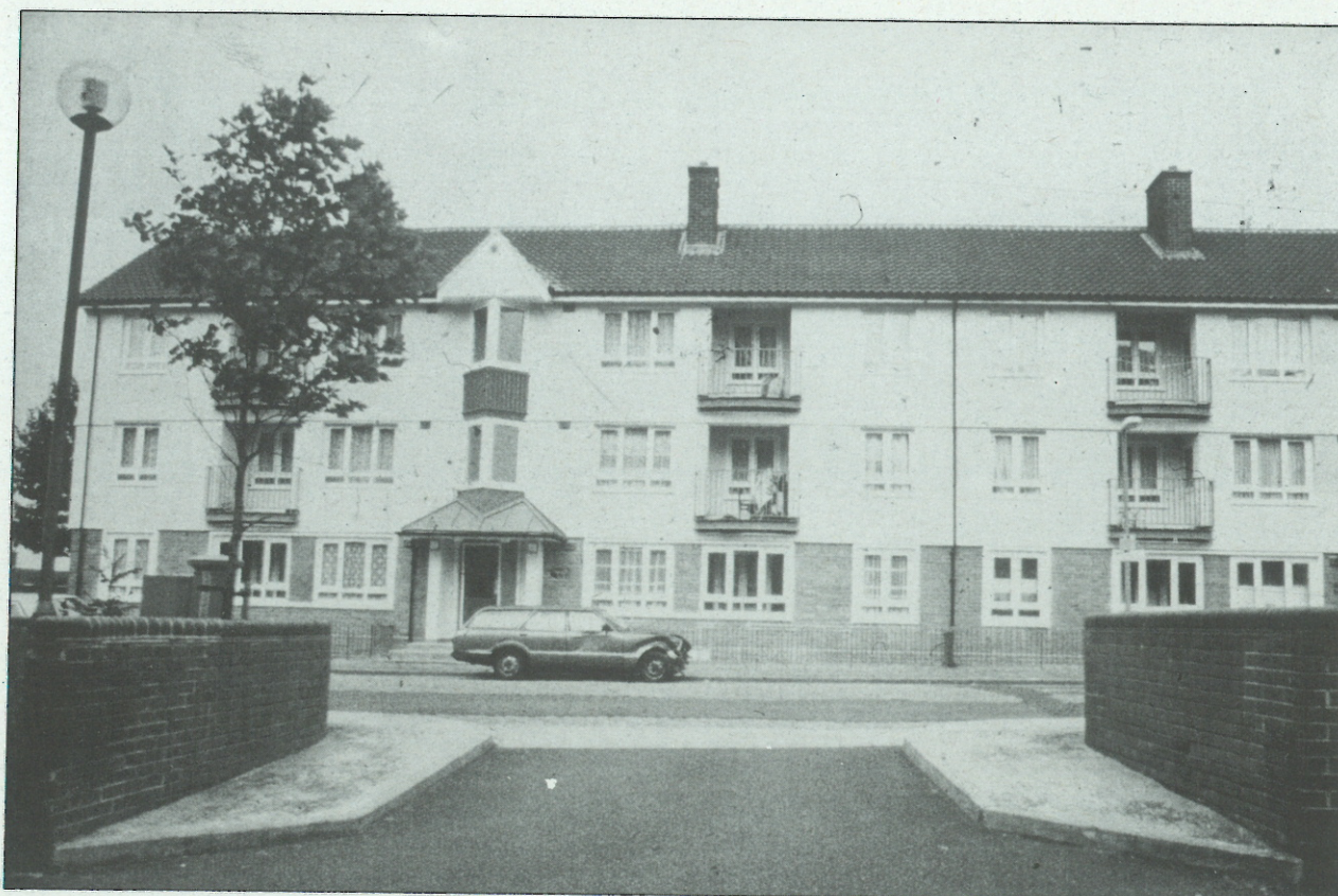
Picture 6: Before and After views of a renovated 1959 block of flats in Estate Action Phase One
